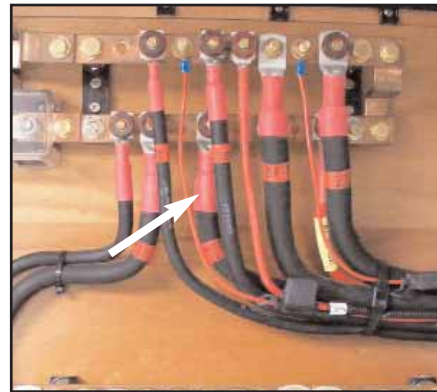
FUSE OF HYDRAULIC SYSTEM (GANGWAY)
