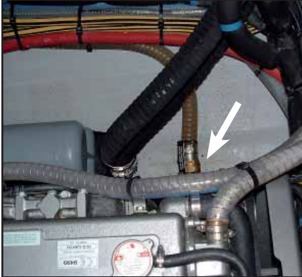
ENGINE WATER SUCTION VALVE
